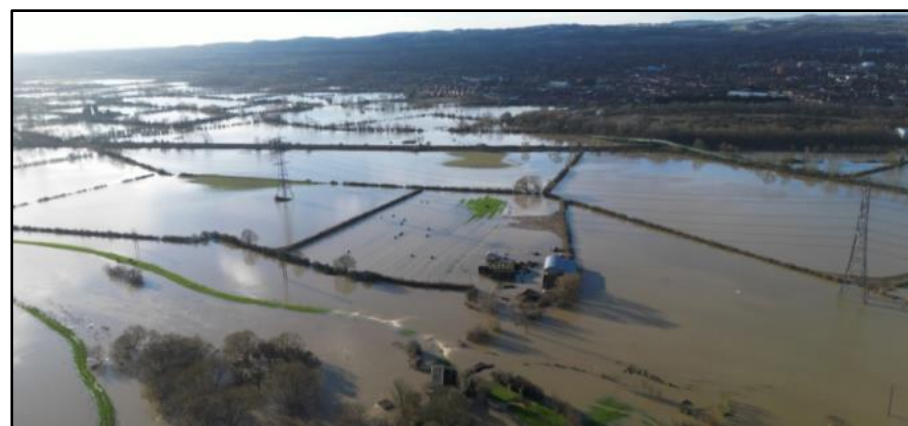
Flooding in Charnwood January 2025
