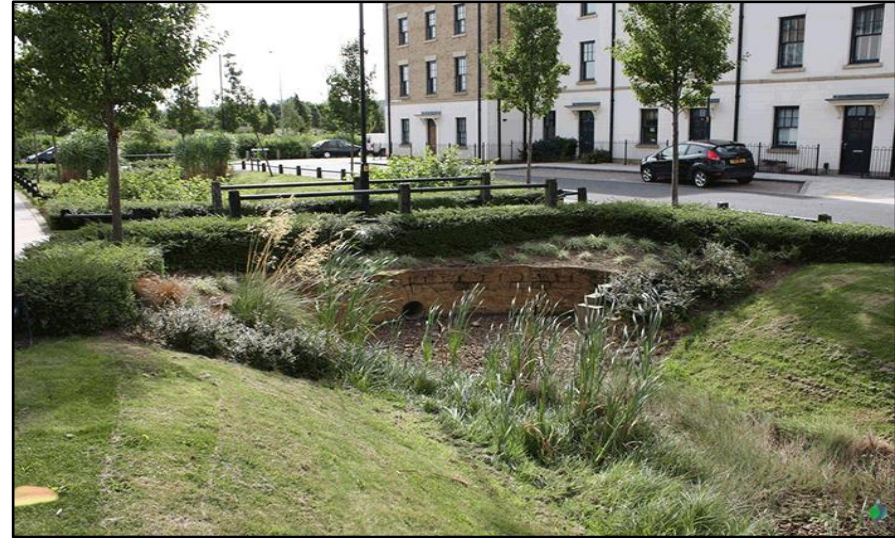
Sustainable Drainage System retrofitted in Mansfield
